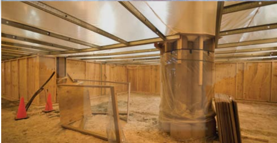
INSET AND BELOW: New granite floor under construction
